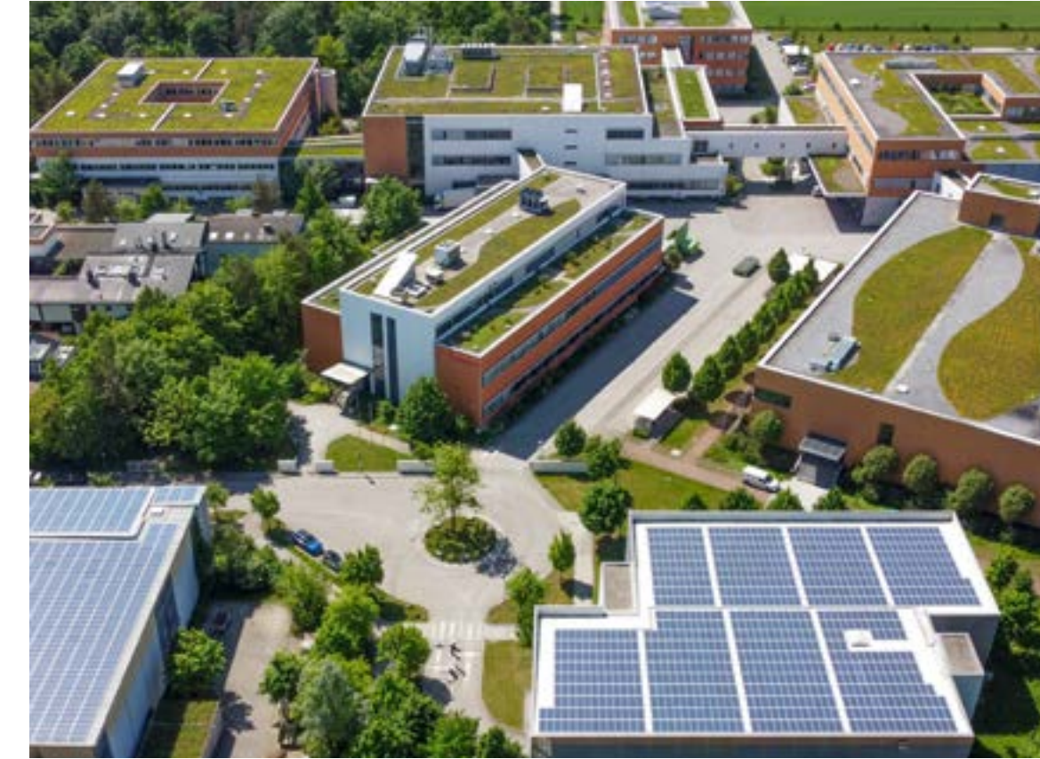
The Schreiner Group Headquarters in Oberschleissheim.
