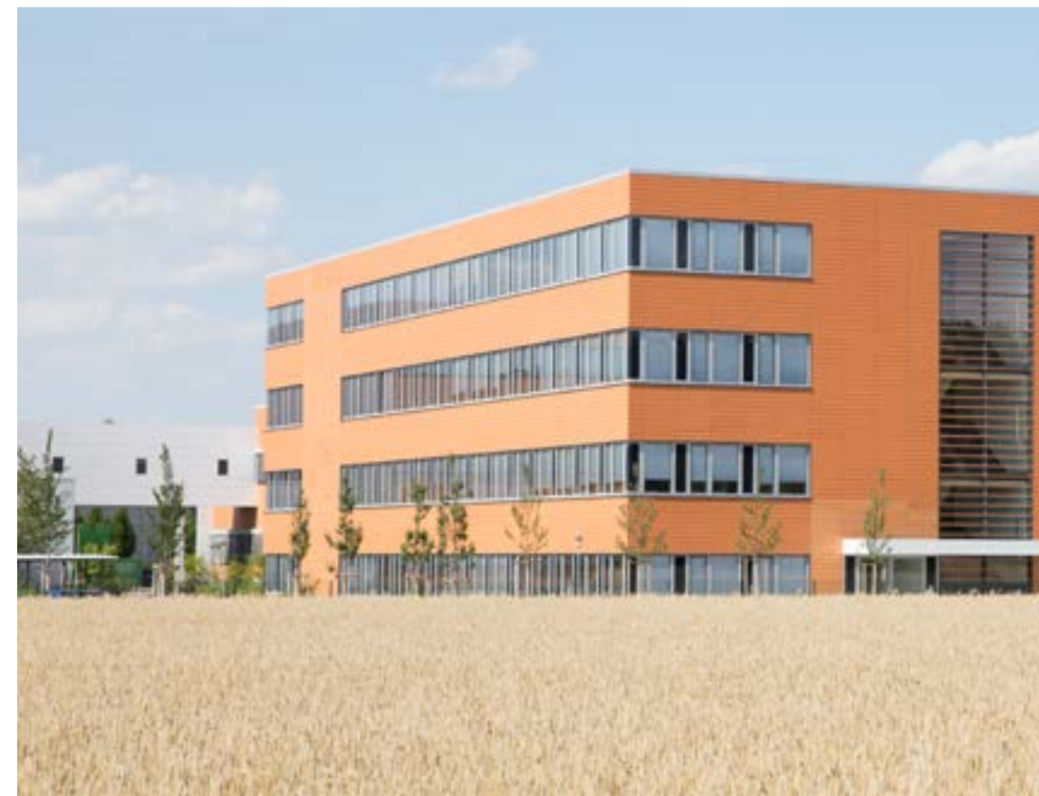
Green building at company headquarters in Oberschleissheim
